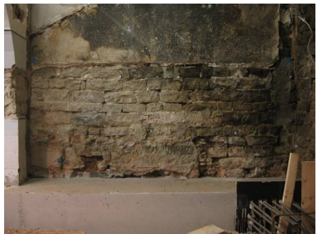
16. Parament interior UE 3088
