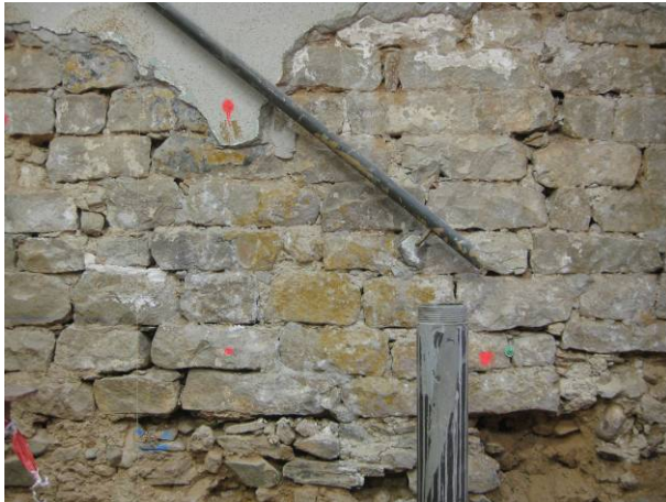
19. Parament interior UE 1102
